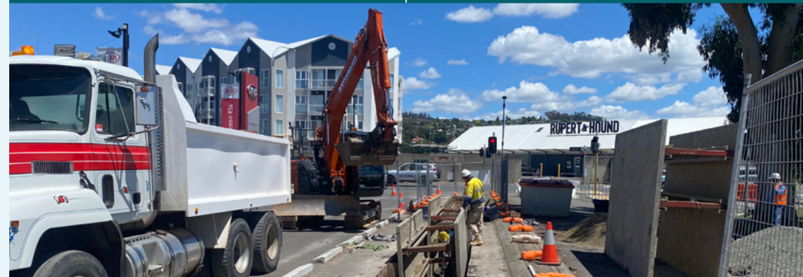
Esplanade/St John Street pipeline works
