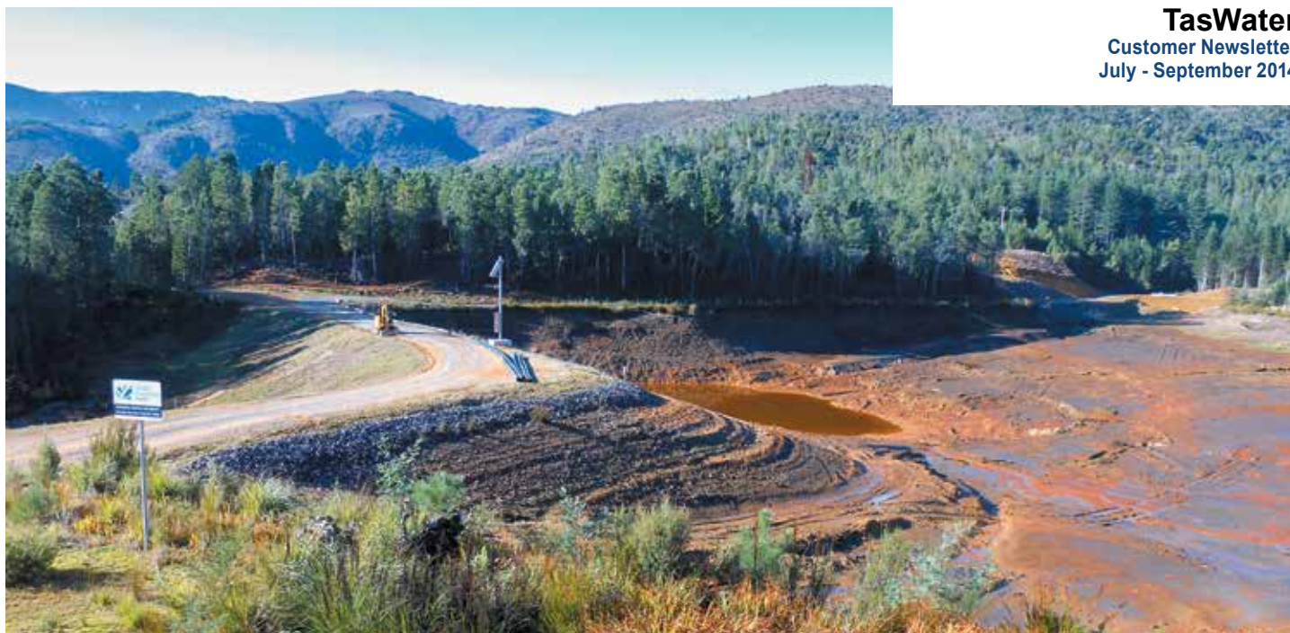
Work is underway to give Queenstown's Conglomerate Dam a facelift
