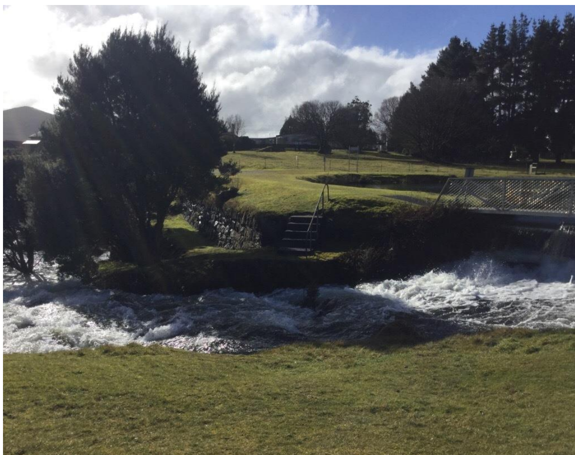
Figure A.4: Upper Pond outlet weir (a) longitudinal profile with 2 m 2 /s discharge and (b) cross section (c) photo
