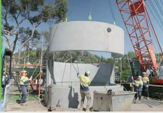
Precast concrete segment lifted into place for the new under-ground diversion chamber at our Margaret Street Pump Station.
