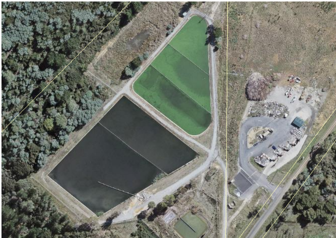
Figure 1-1: Beaconsfield Sewage Treatment Plant
