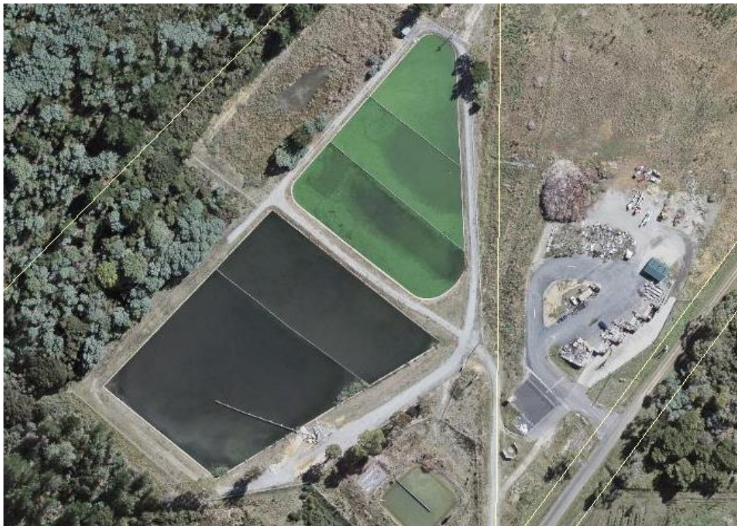
Figure 1-1: Beaconsfield Sewage Treatment Plant
