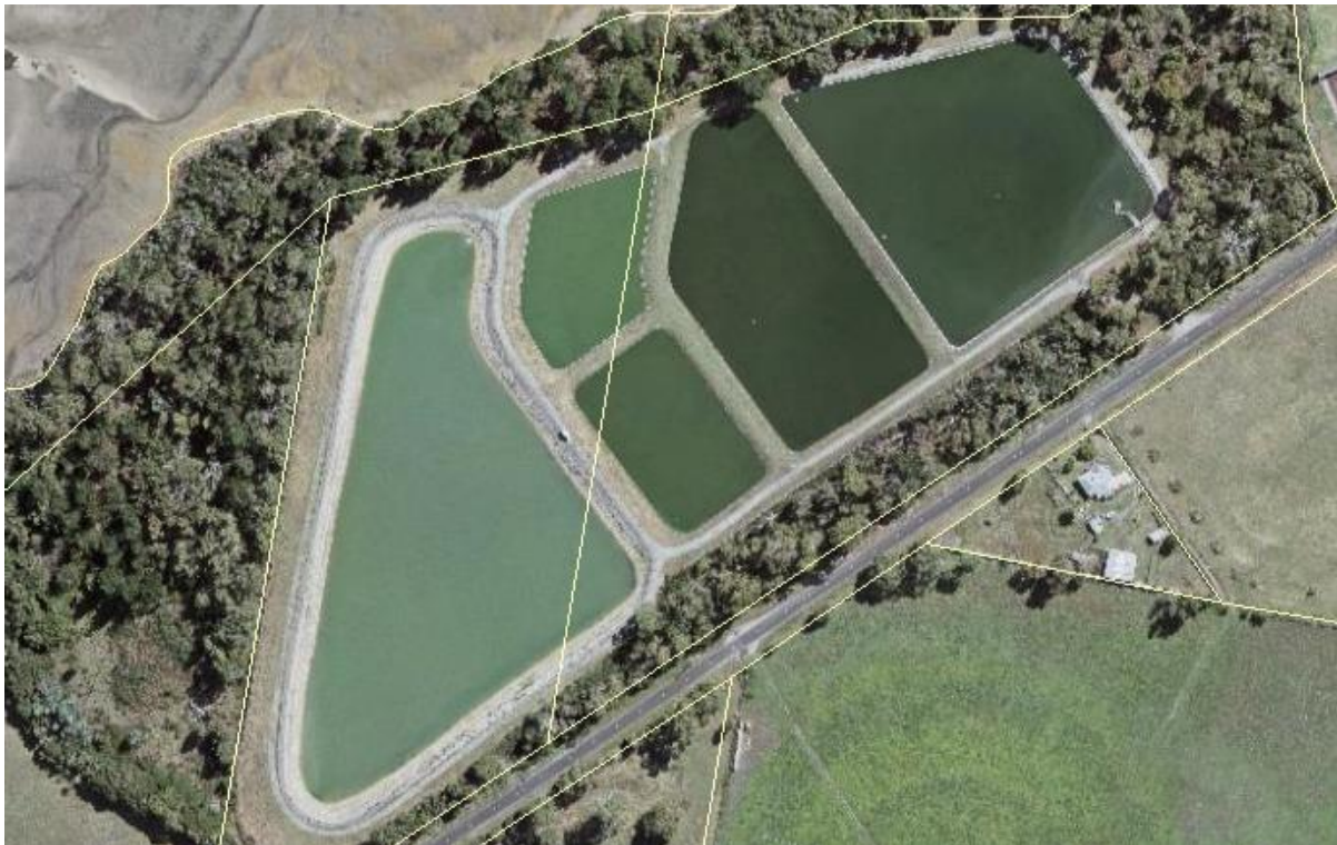
Figure 2-1: Beauty Point Sewage Treatment Plant
