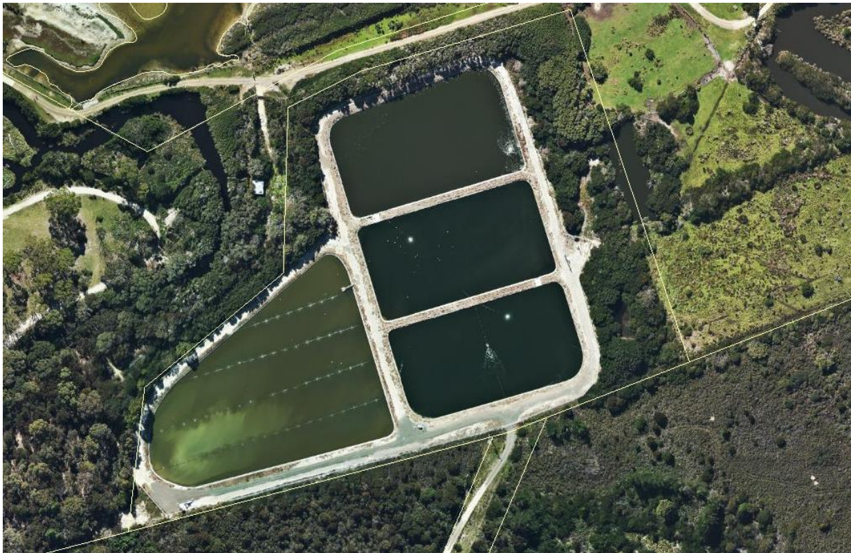
Figure 3-1: Bicheno Sewage Treatment Plant
