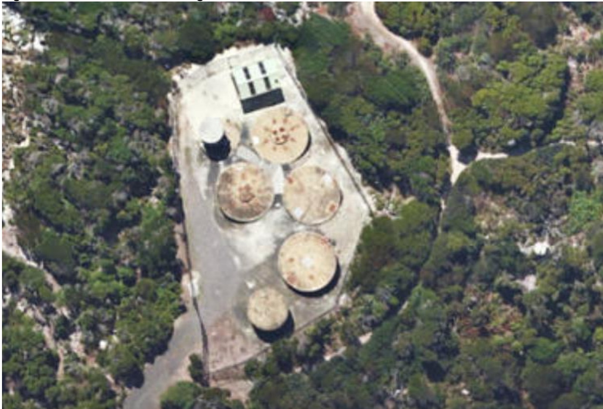
Figure 5-1: Boat Harbour Sewage Treatment Plant
