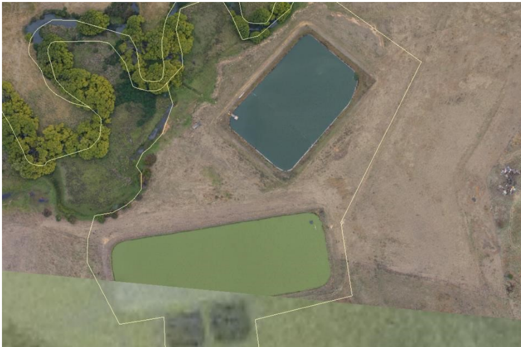
Figure 6-1: Bothwell Sewage Treatment Plant
