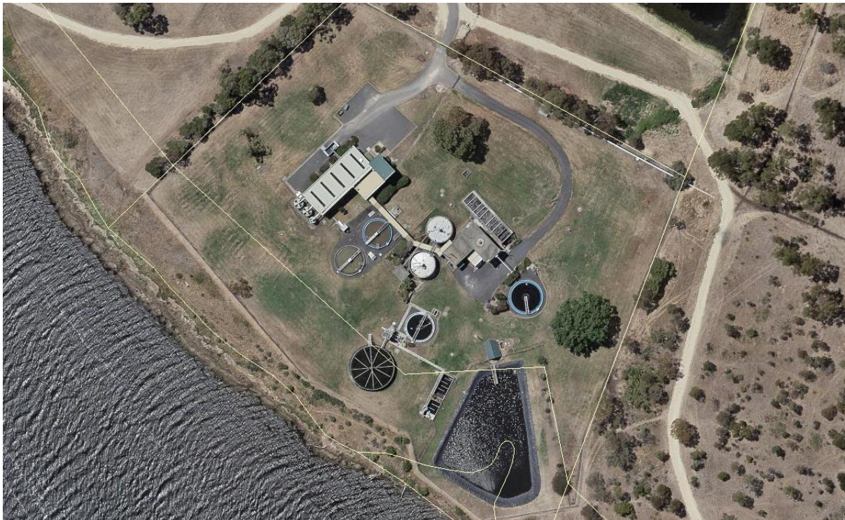
Figure 26–1: Green Point Sewage Treatment Plant
