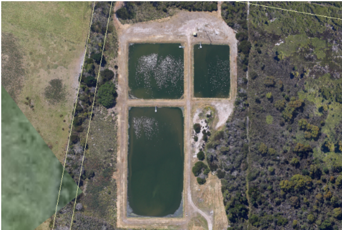
Figure 7-1: Bridport Sewage Treatment Plant
