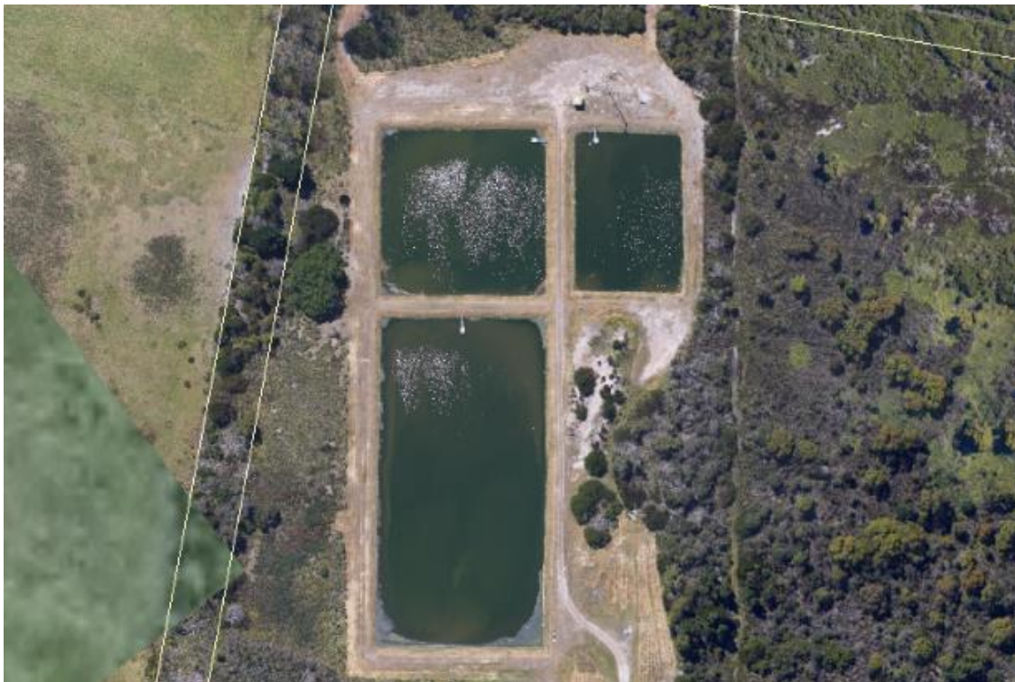
Figure 7-1: Bridport Sewage Treatment Plant
