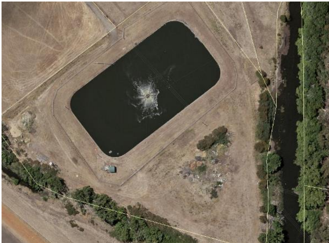
Figure 8-1: Brighton Sewage Treatment Plant
