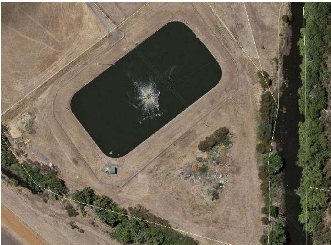
Figure 8-1: Brighton Sewage Treatment Plant
