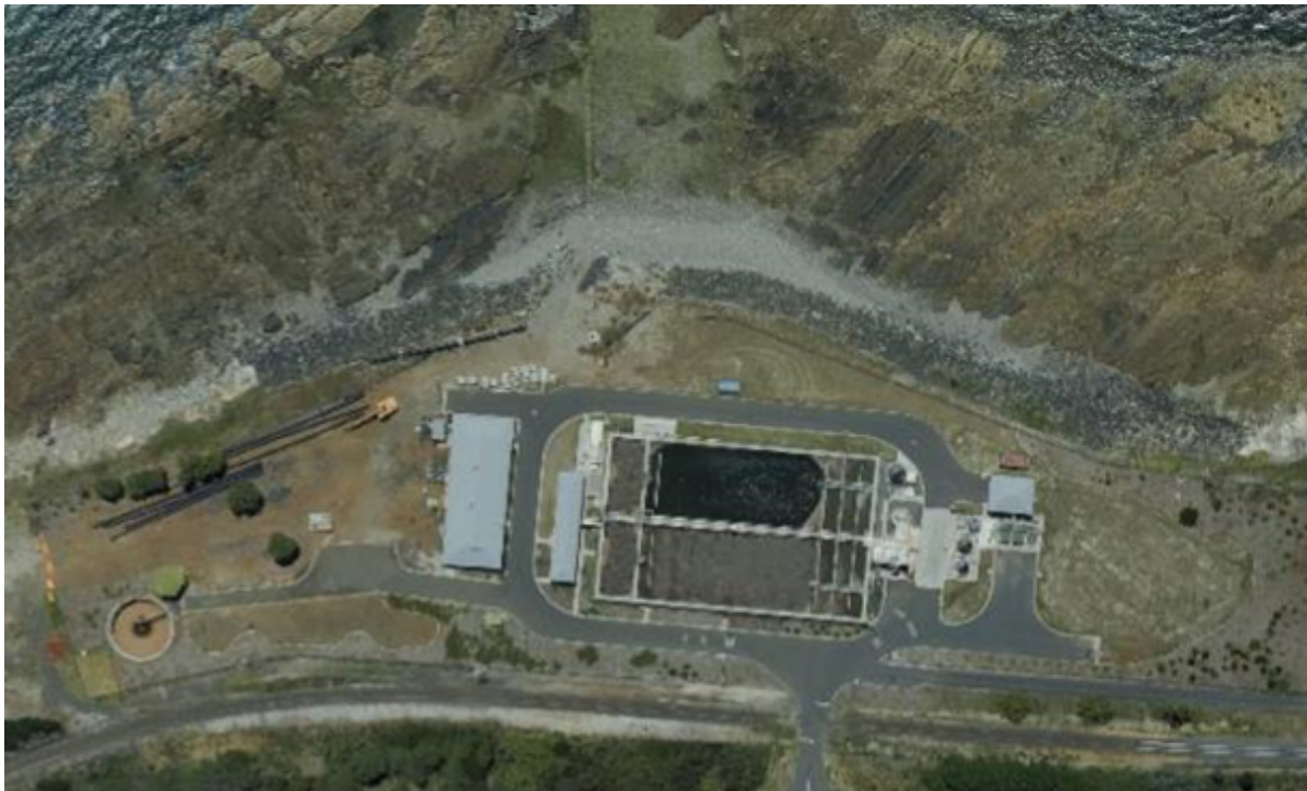
Figure 9–1: Round Hill (Burnie) Sewage Treatment Plant
