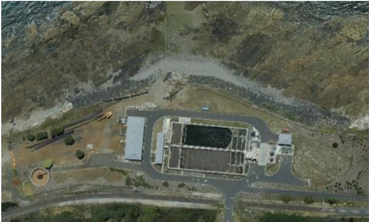
Figure 9-1: Round Hill (Burnie) Sewage Treatment Plant
