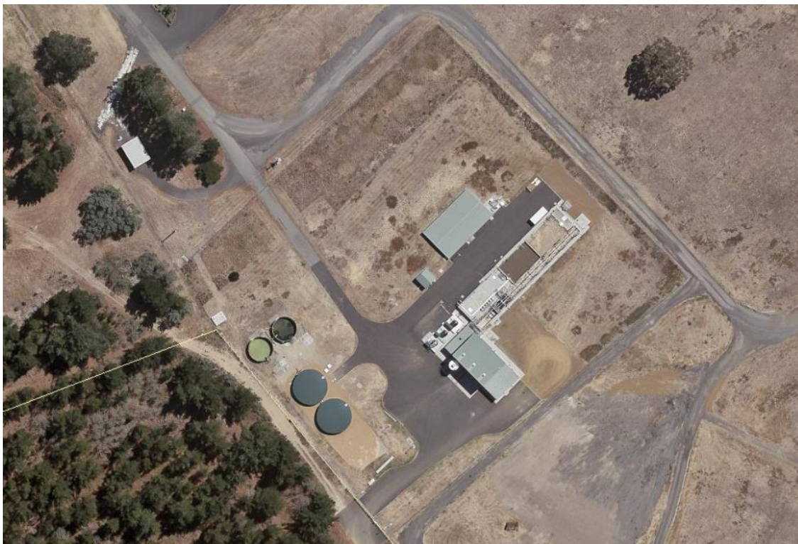
Figure 10-1: Cambridge Sewage Treatment Plant
