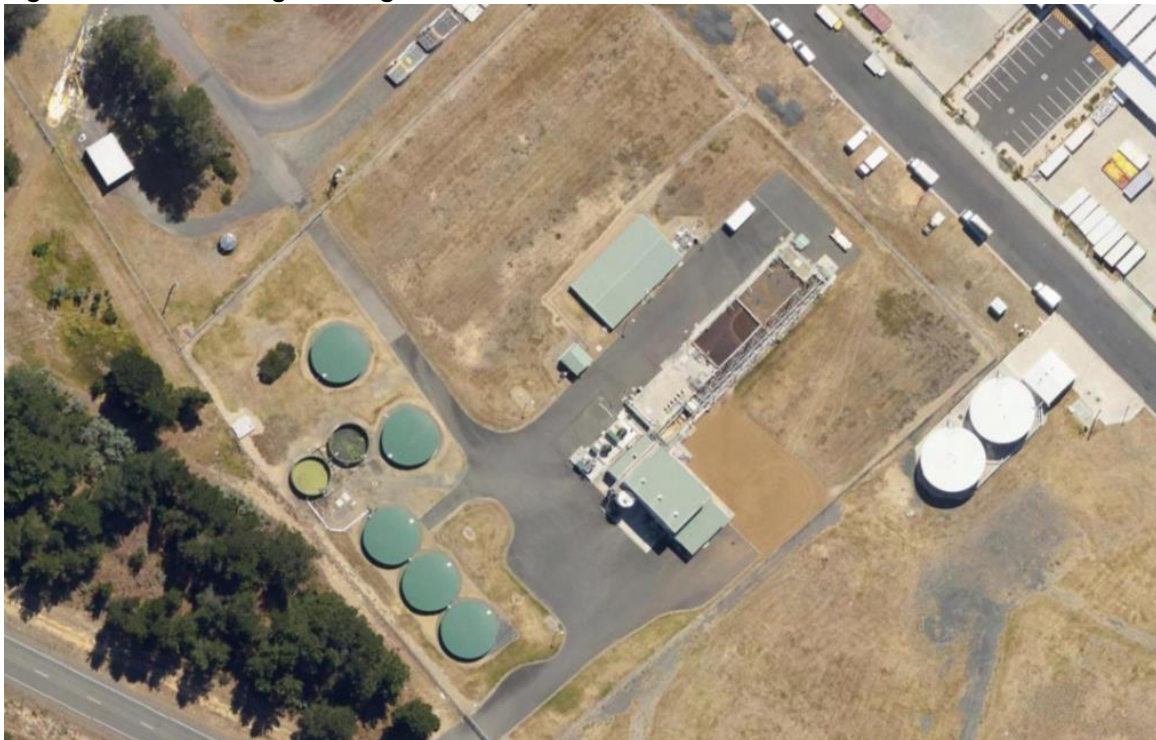
Figure 10-1: Cambridge Sewage Treatment Plant
