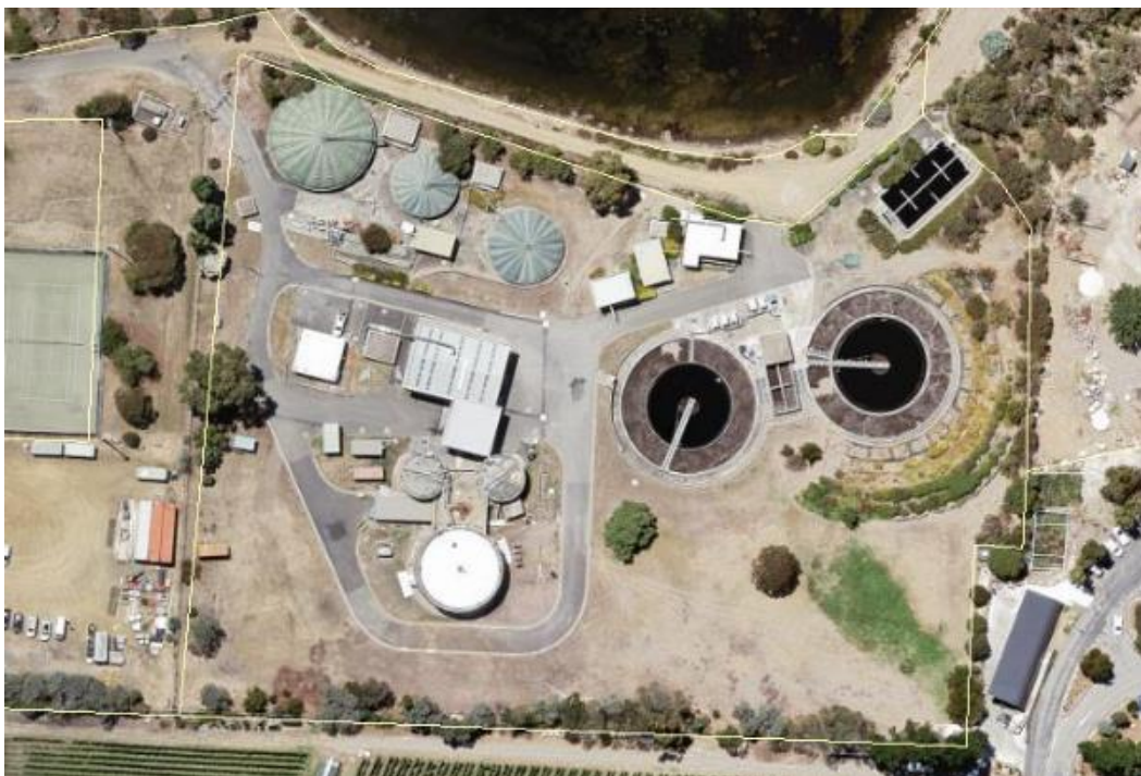
Figure 11-1: Cameron Bay Sewage Treatment Plant
