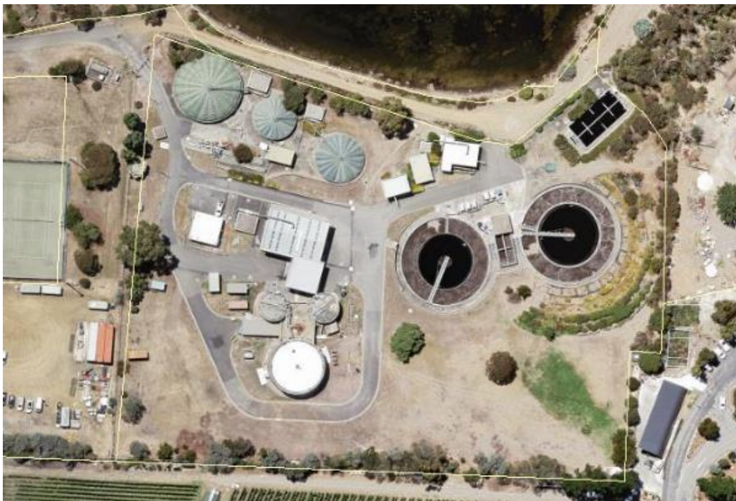
Figure 11-1: Cameron Bay Sewage Treatment Plant
