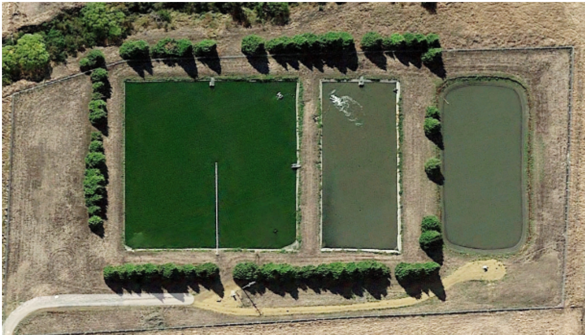
Figure 12-1: Campania Sewage Treatment Plant
