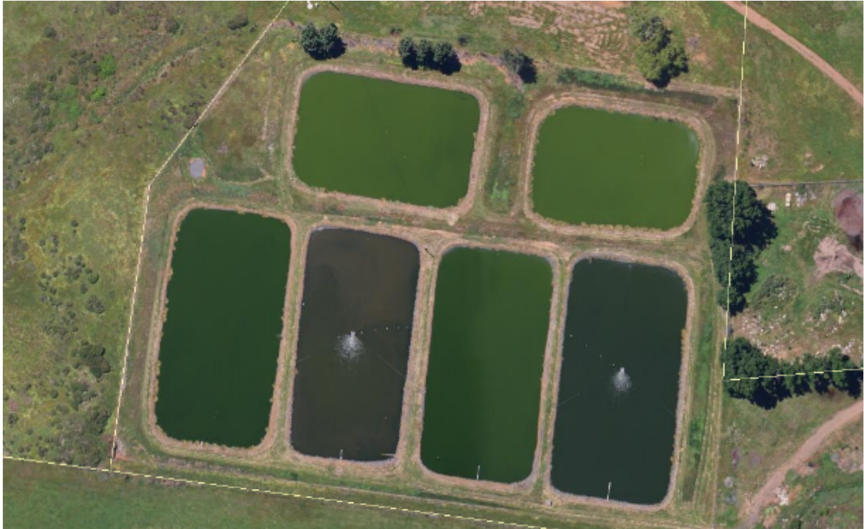
Figure 13-1: Campbell Town Sewage Treatment Plant
