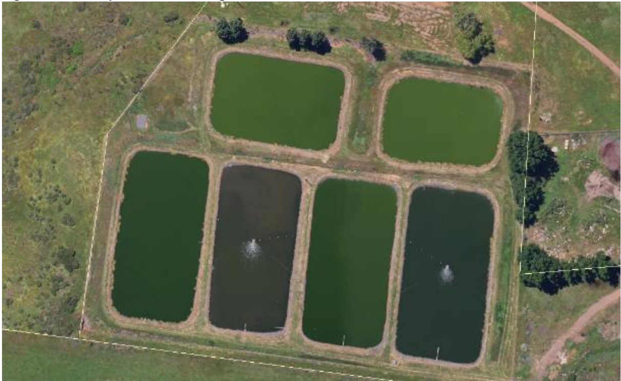
Figure 13-1: Campbell Town Sewage Treatment Plant
