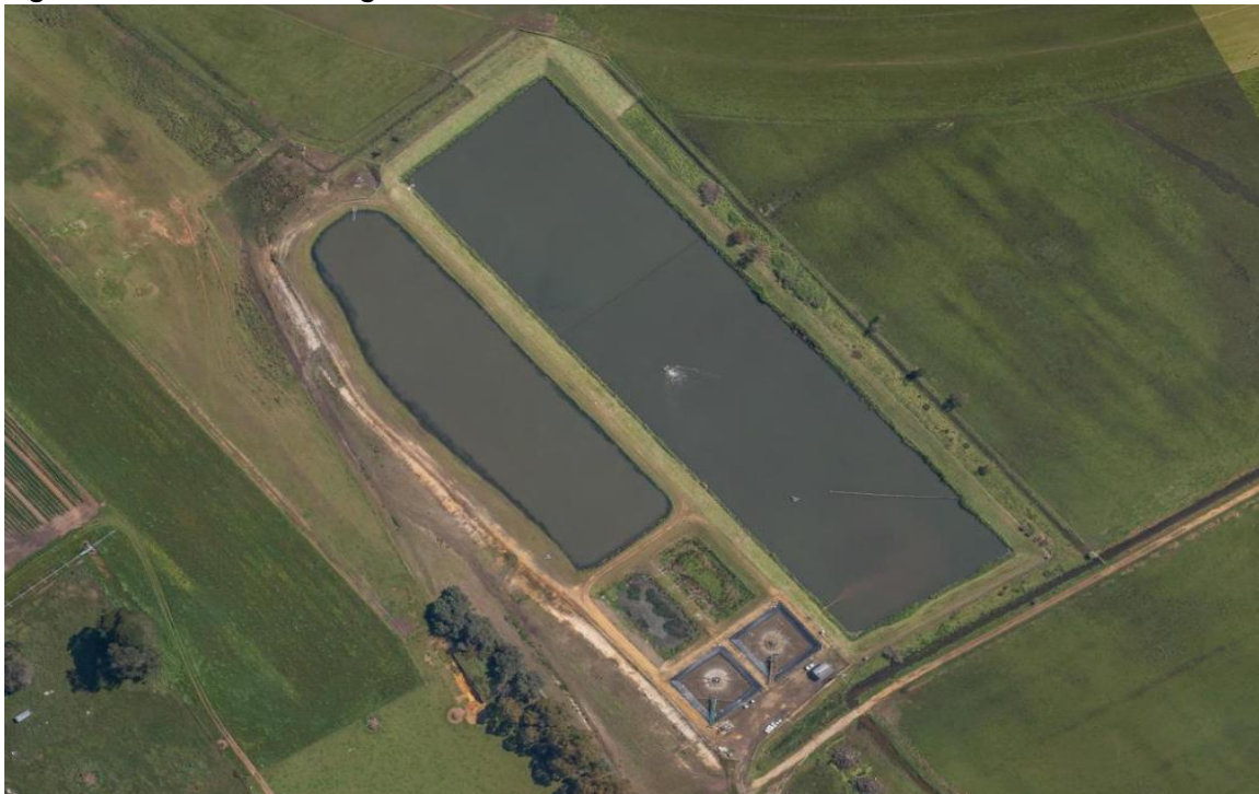
Figure 14-1: Carrick Sewage Treatment Plant
