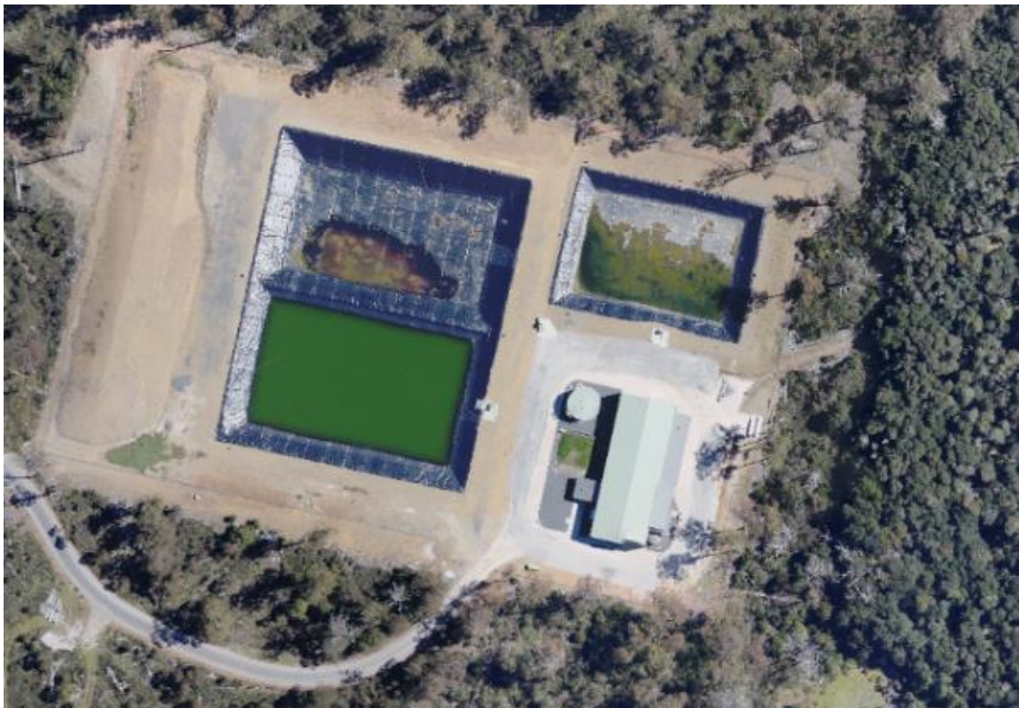
Figure 15-1: Cradle Valley Sewage Treatment Plant
