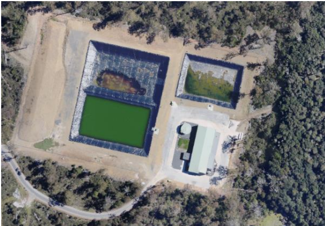
Figure 15-1: Cradle Valley Sewage Treatment Plant
