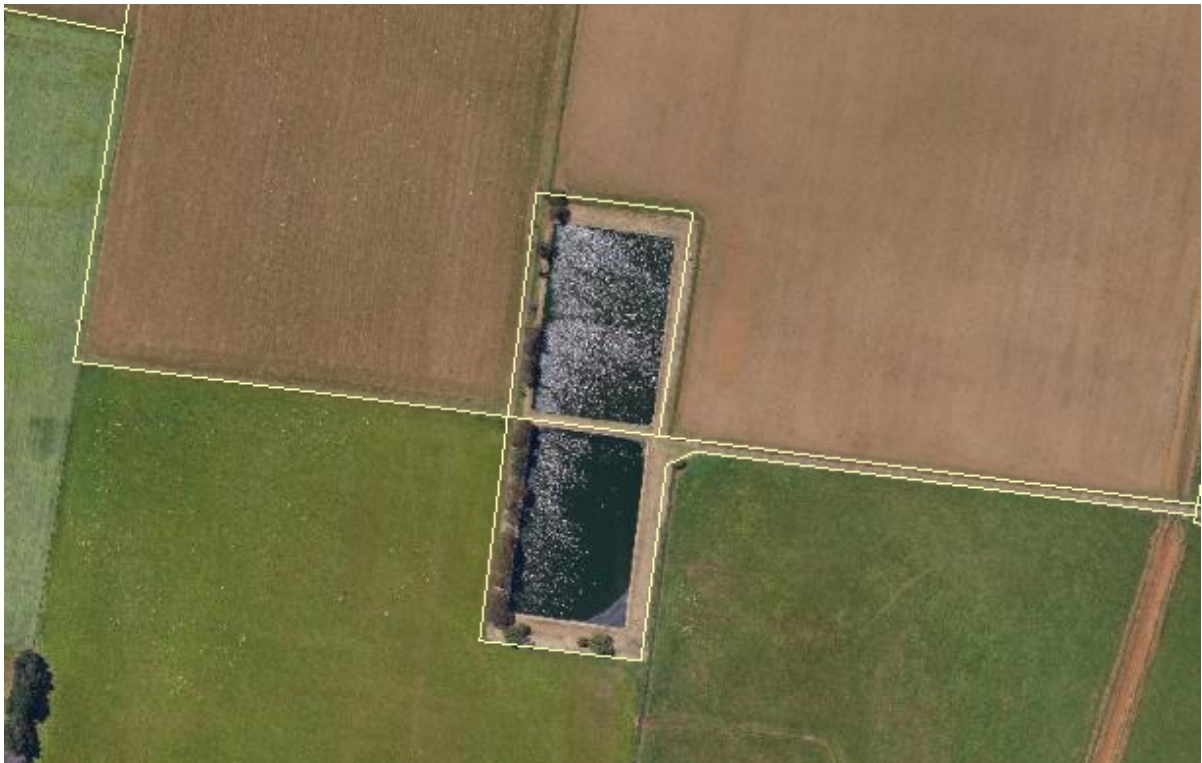
Figure 16-1: Cressy Sewage Treatment Plant
