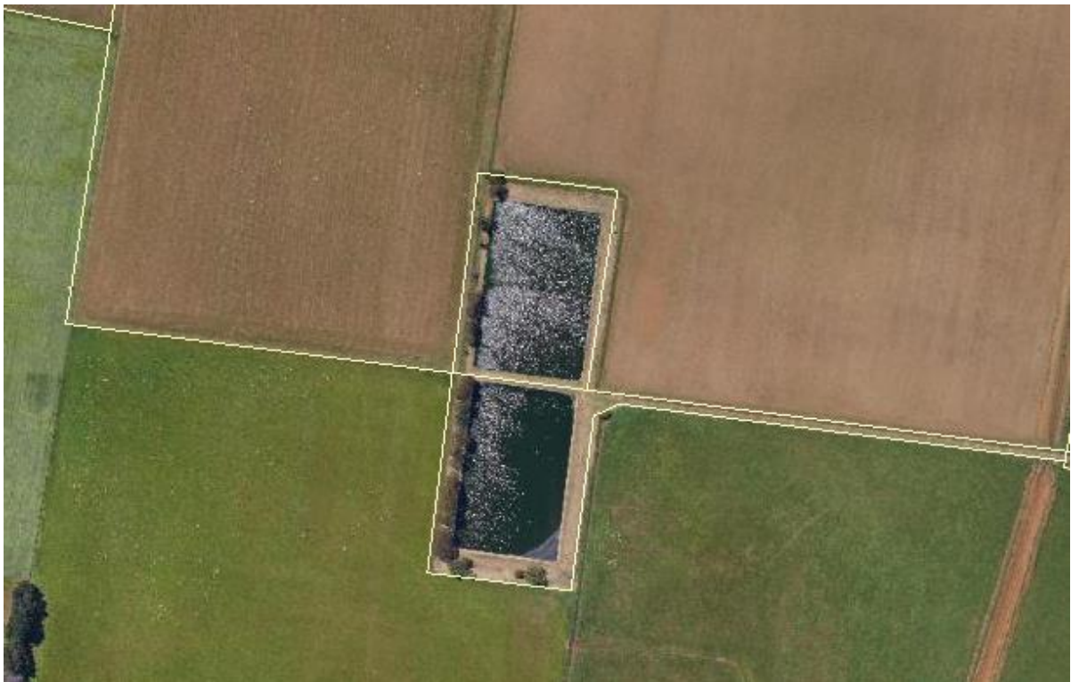
Figure 16-1: Cressy Sewage Treatment Plant
