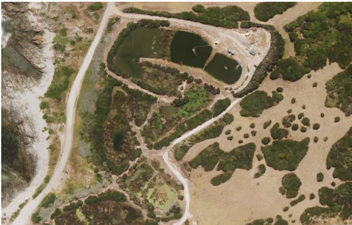
Figure 17-1: Currie Sewage Treatment Plant
