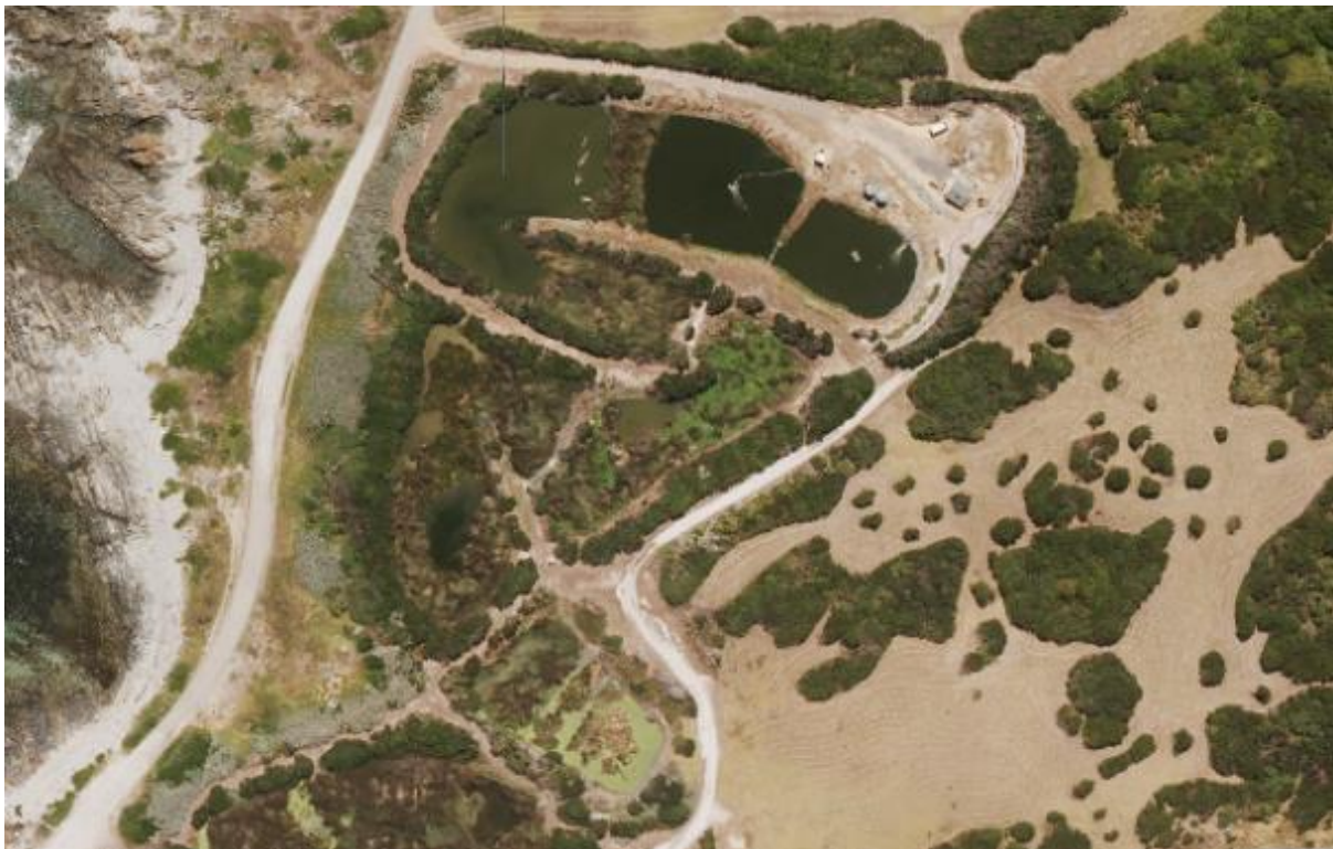
Figure 17-1: Currie Sewage Treatment Plant
