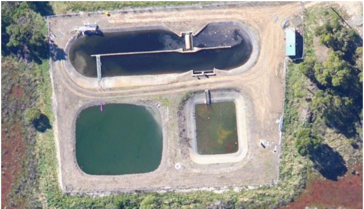
Figure 18-1: Cygnet Sewage Treatment Plant
