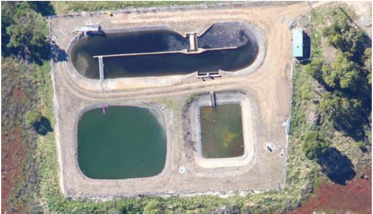
Figure 18-1: Cygnet Sewage Treatment Plant
