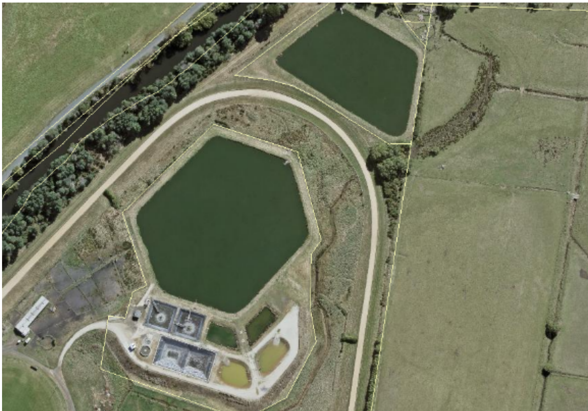
Figure 19-1: Deloraine Sewage Treatment Plant
