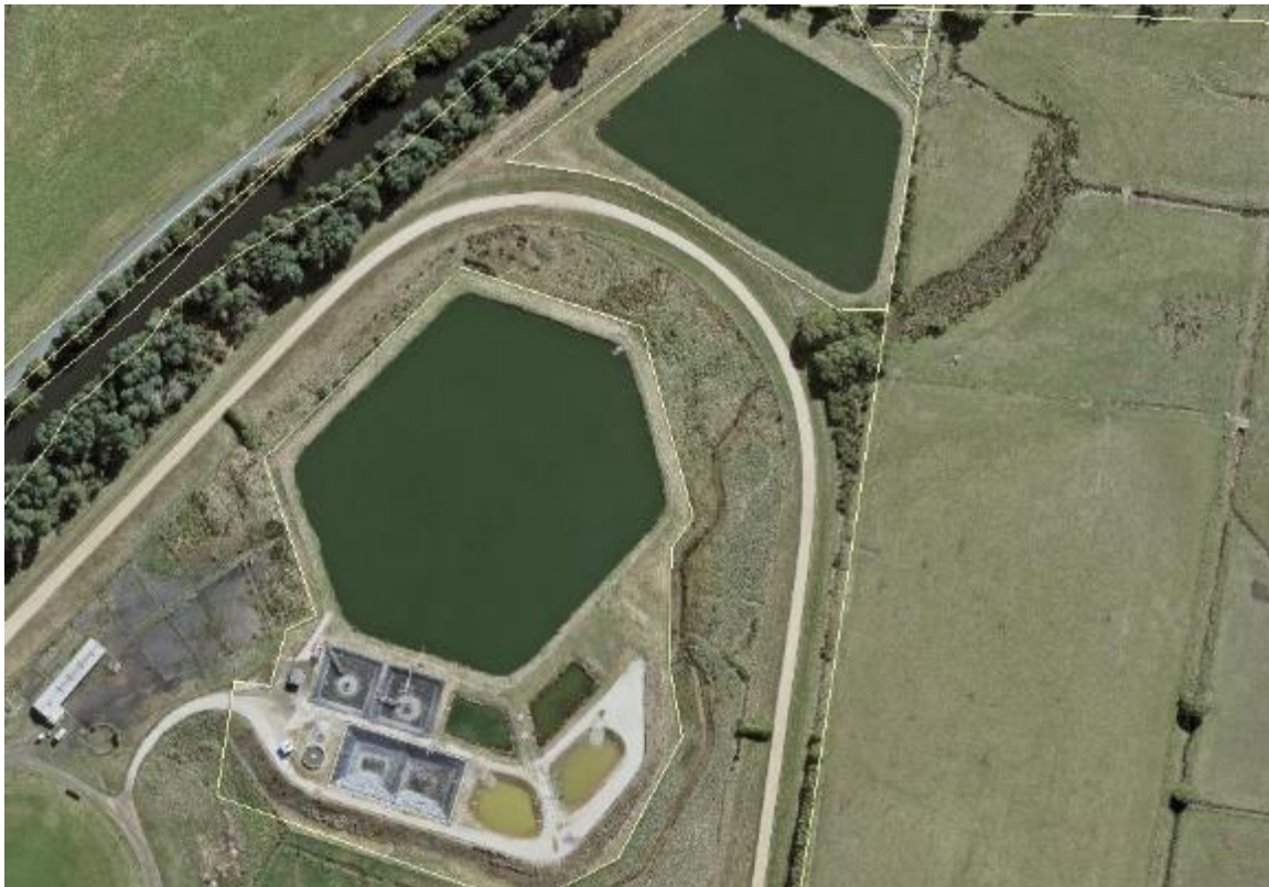
Figure 19-1: Deloraine Sewage Treatment Plant
