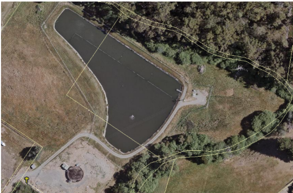
Figure 20–1: Dover Sewage Treatment Plant
