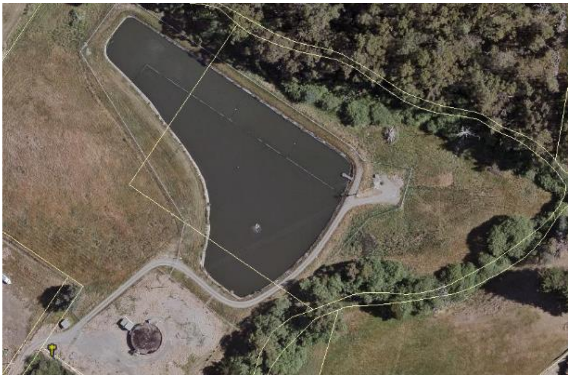
Figure 20–1: Dover Sewage Treatment Plant
