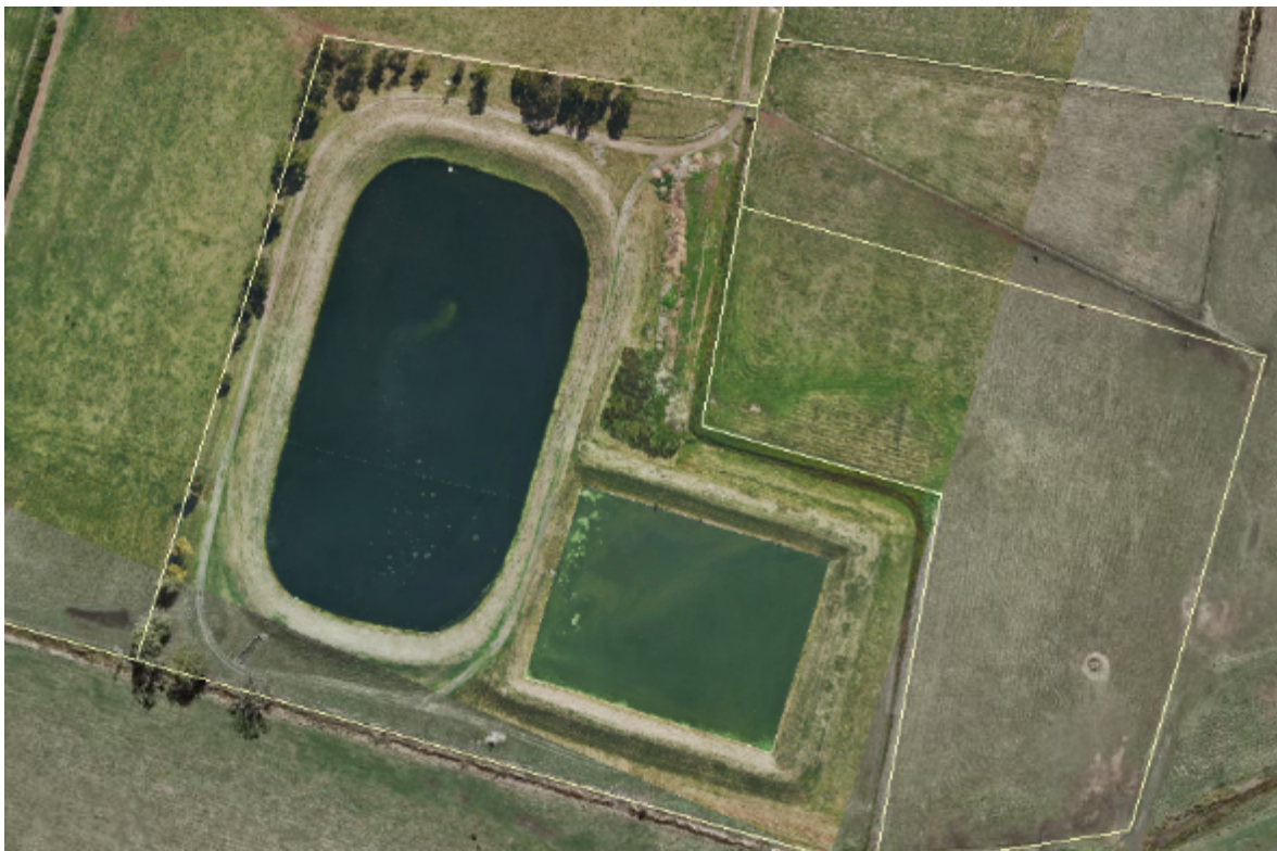
Figure 21-1: Evandale Sewage Treatment Plant
