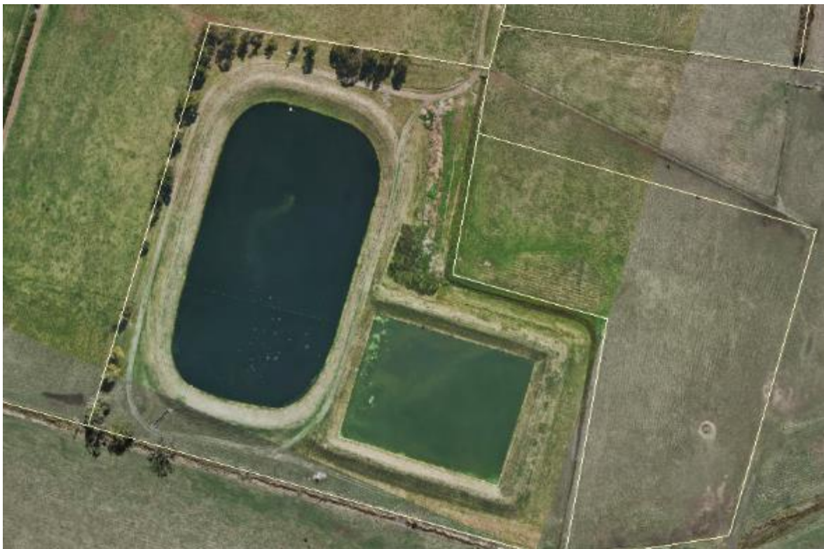
Figure 21-1: Evandale Sewage Treatment Plant
