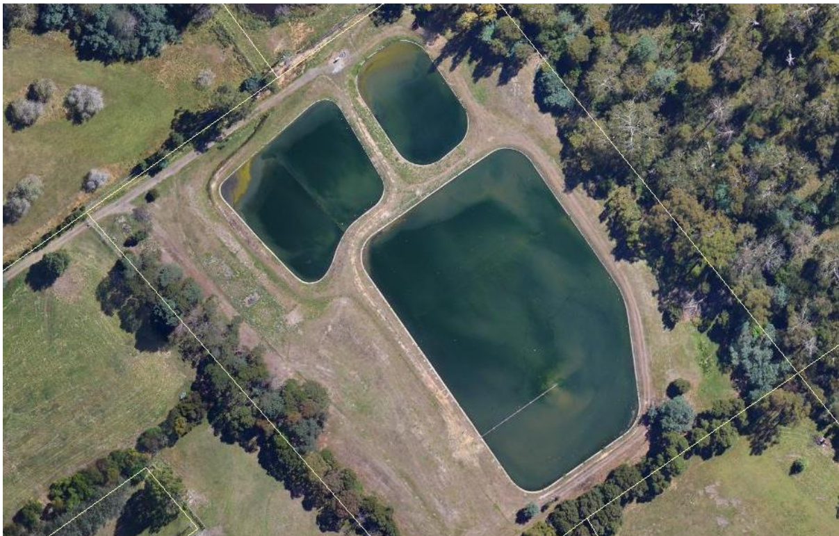
Figure 22-1: Exeter Sewage Treatment Plant
