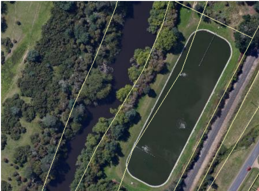
Figure 23-1: Fingal Sewage Treatment Plant
