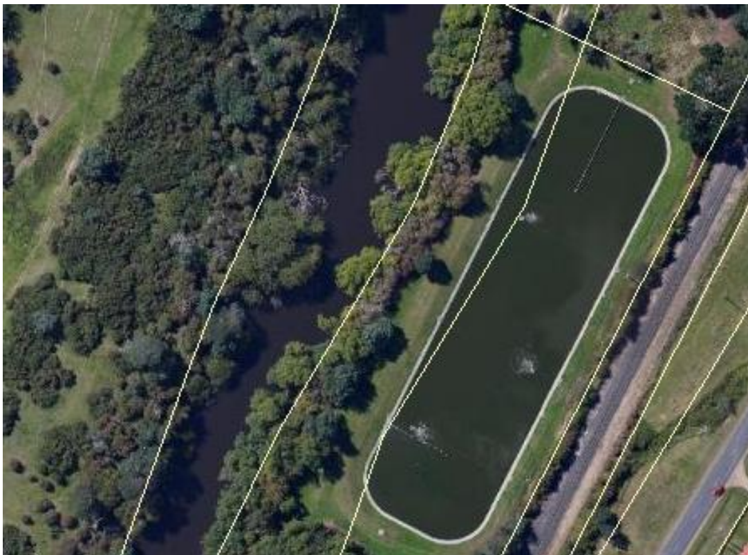
Figure 23-1: Fingal Sewage Treatment Plant
