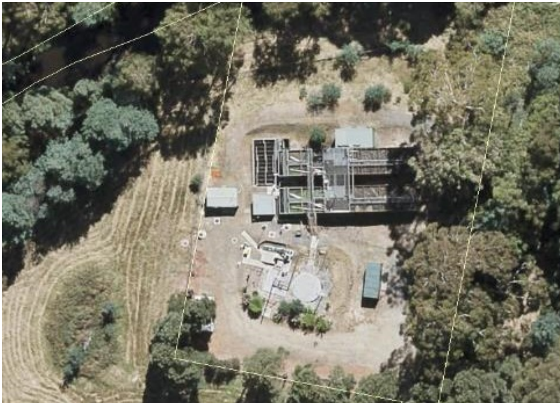
Figure 24-1: Geeveston Sewage Treatment Plant
