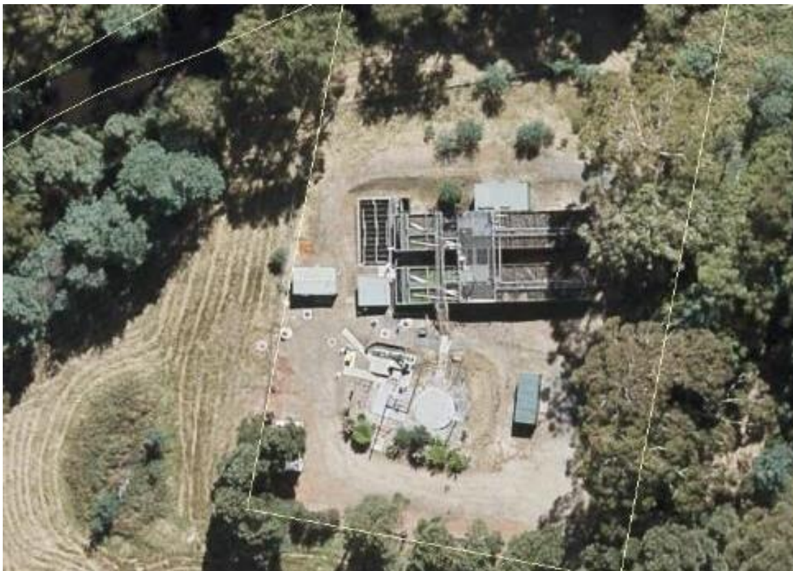
Figure 24-1: Geeveston Sewage Treatment Plant
