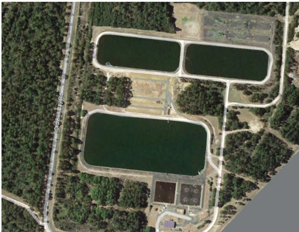
Figure 25-1: George Town Sewage Treatment Plant
