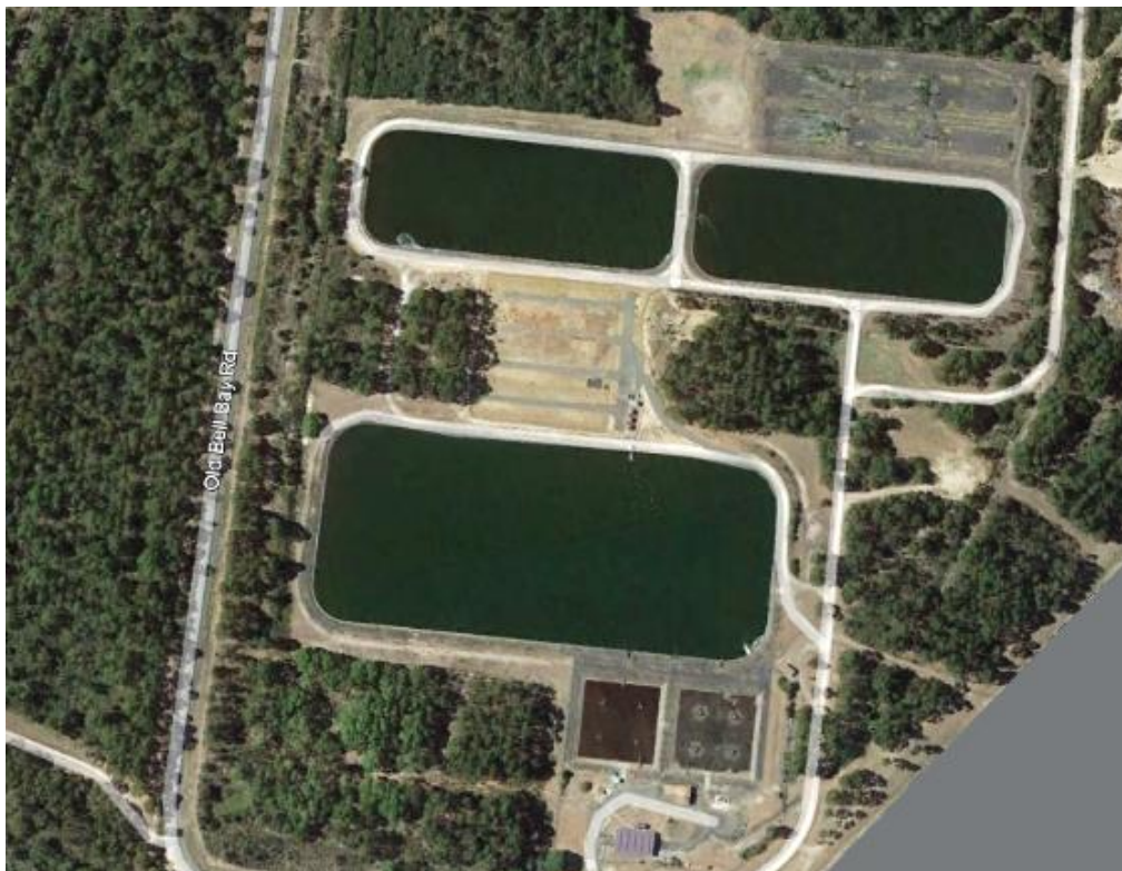
Figure 25-1: George Town Sewage Treatment Plant
