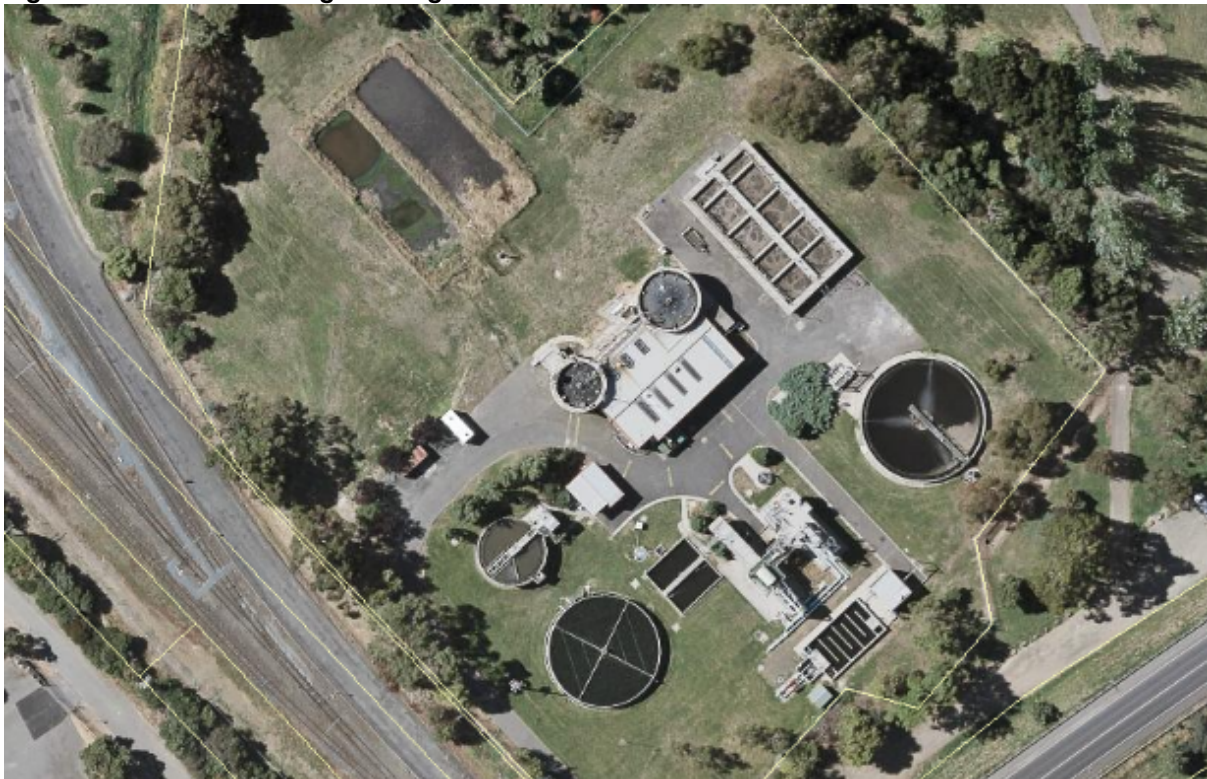
Figure 27-1: Hoblers Bridge Sewage Treatment Plant
