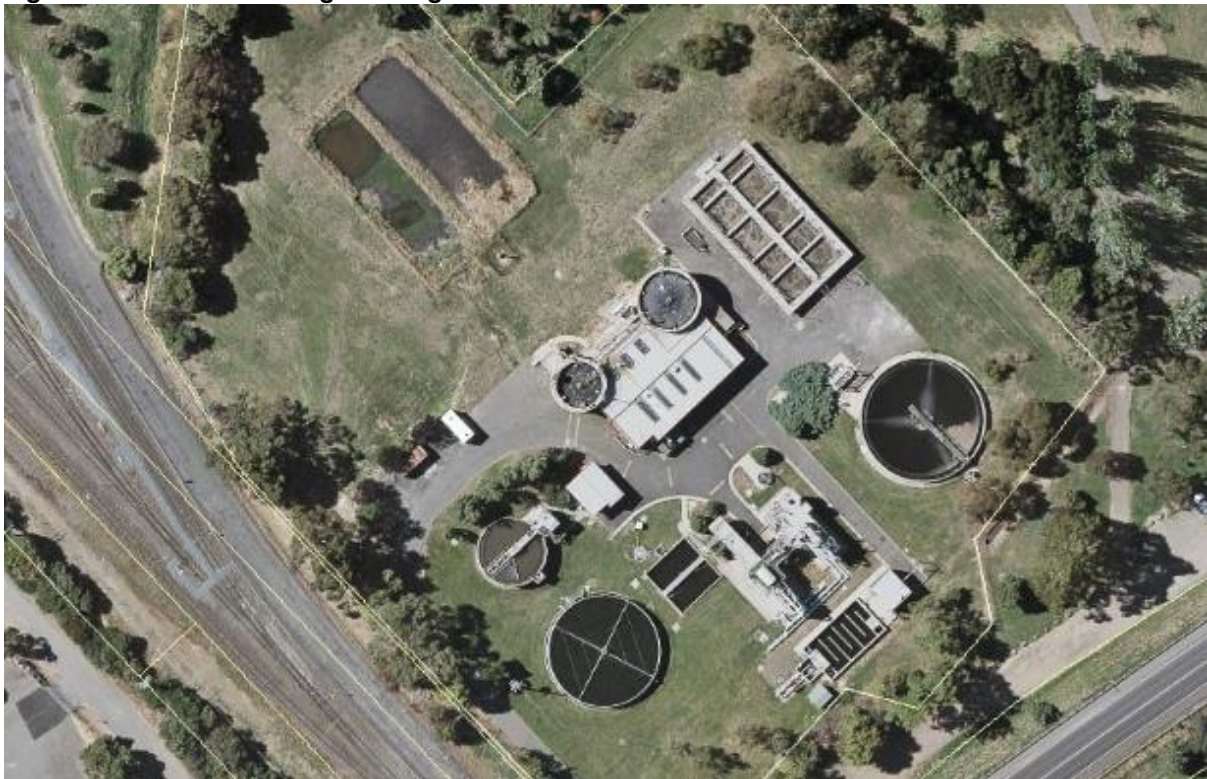
Figure 27-1: Hoblers Bridge Sewage Treatment Plant
