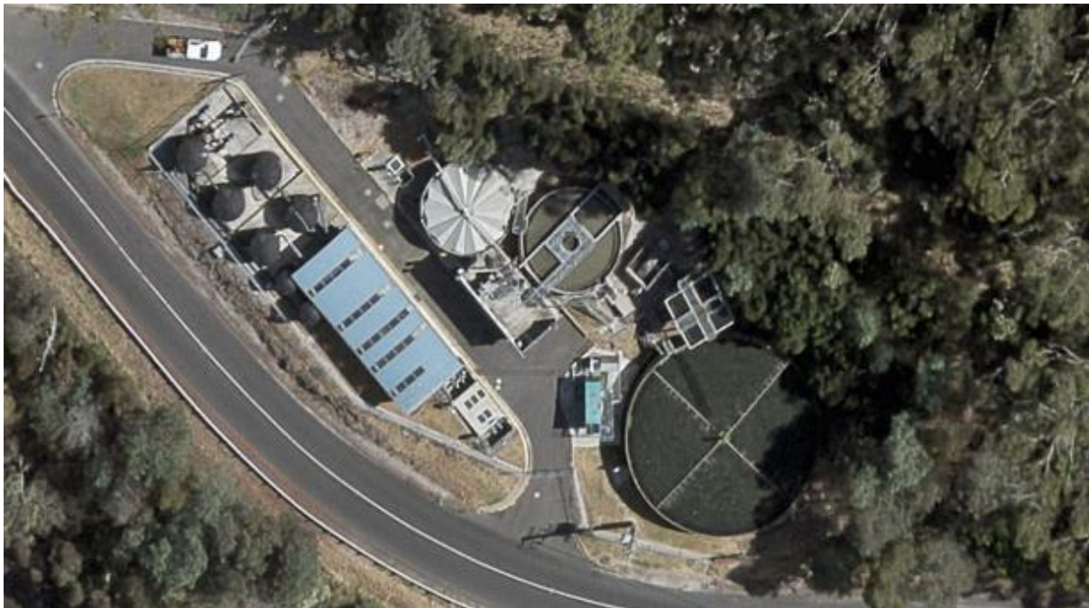
Figure 29-1: Latrobe Sewage Treatment Plant
