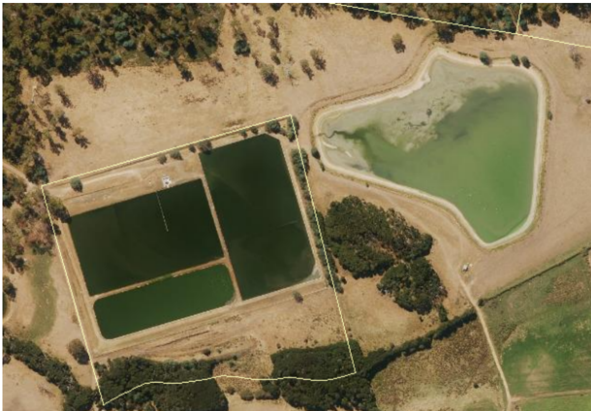
Figure 30–1: Legana Sewage Treatment Plant
